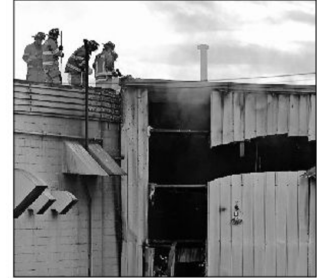
Firefighters work at the scene of a factory fire Monday in New Windsor, N.Y. Two explosions and a fire at a cosmetics factory about an hour's drive north of New York City left 30 to 35 people injured, including seven firefighters caught in the second blast, authorities said Monday. The first explosion occurred about 10:15 a.m. Monday at the Verla International cosmetics factory, New Windsor police said. (SETH WENIG/THE ASSOCIATED PRESS)
