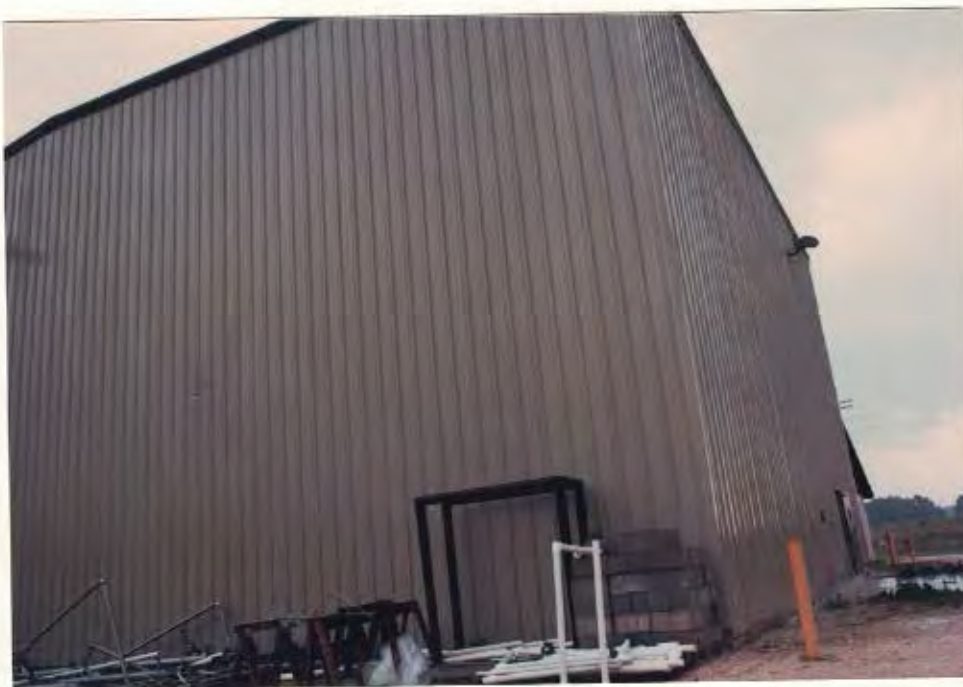
REAR AND SOUTH SIDE OF SUBJECT
