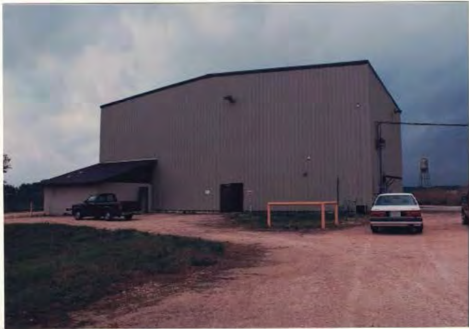
FRONT VIEW OF SUBJECT BOILER ROOM EXTENSION AT LEFT
