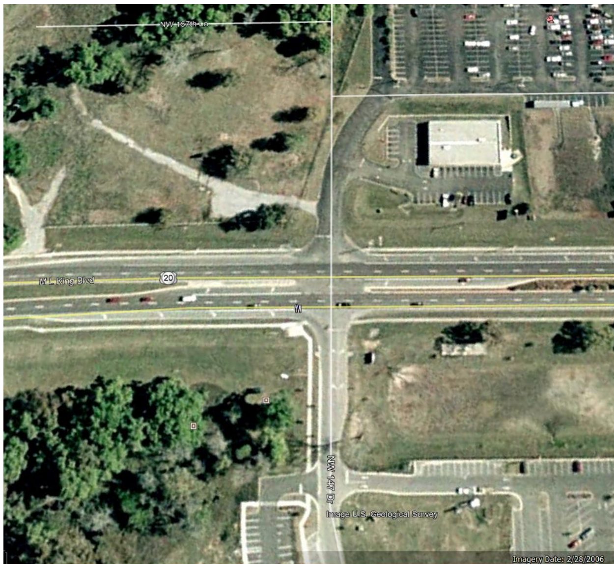
Figure 11 | February 2006 Aerial of US HWY 441 at NW 147 th Drive
