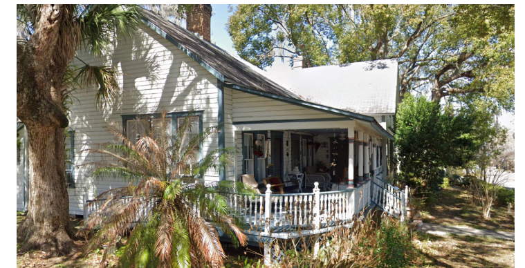
2: Structure: Lean-to Porch Roof 14712 Main St
