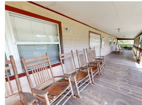
EXISTING OUTDOOR PORCH
