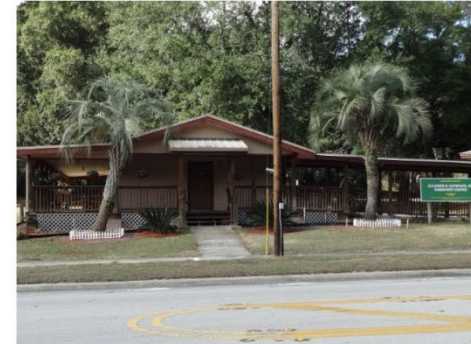
EXISTING HATHCOCK CENTER BUILDING
