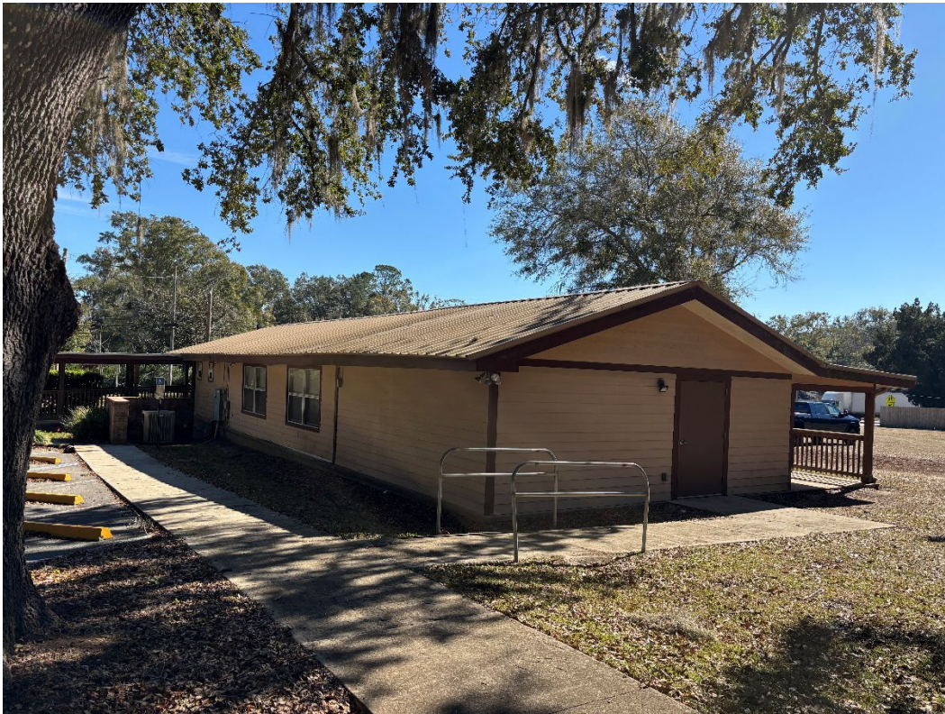
Photograph 2: Overview of north & west elevations
