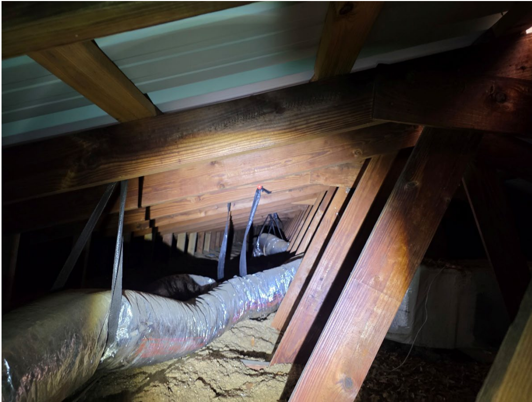
Photograph 4: Example of the roof trusses
