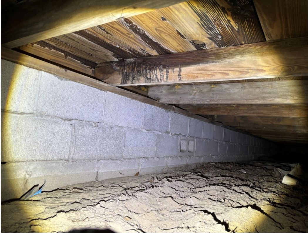
Photograph 7: Example of floor framing bearing on CMU stem wall
