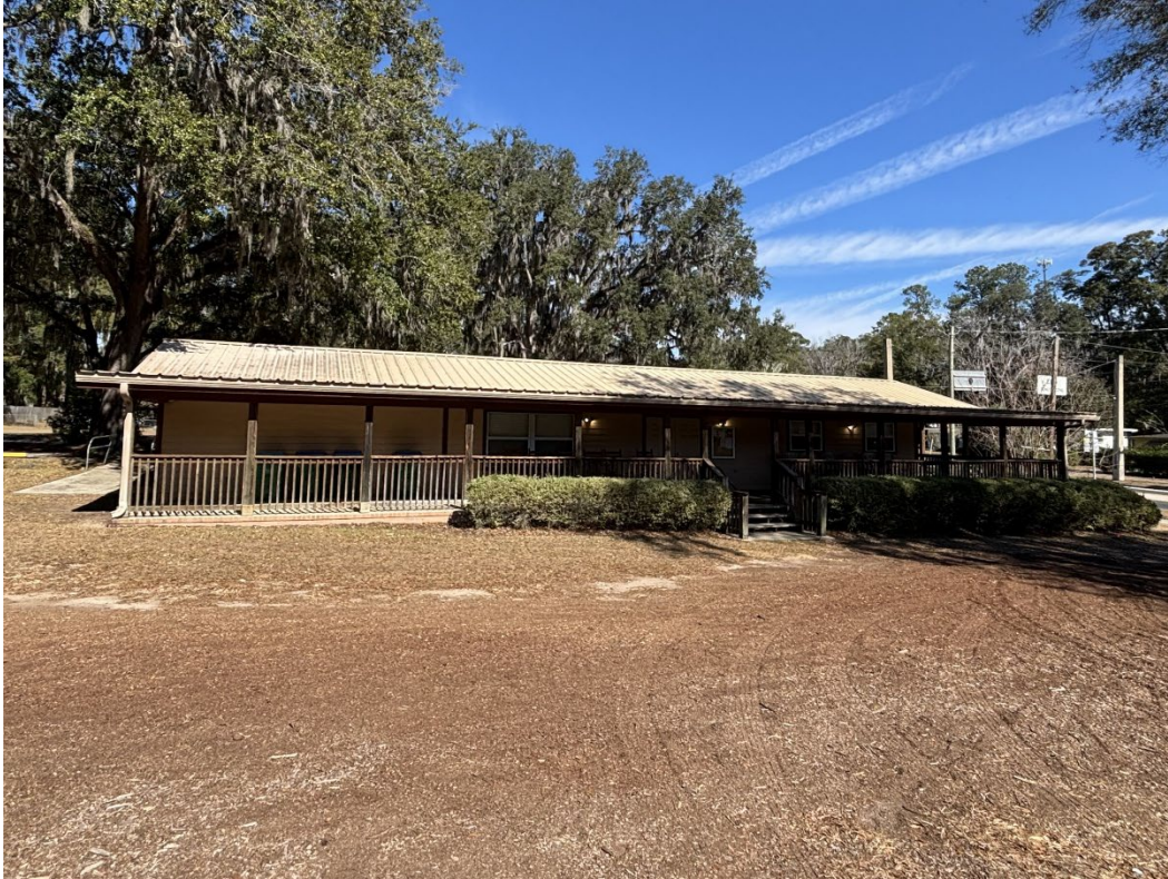
Photograph 1: Overview of south elevation
