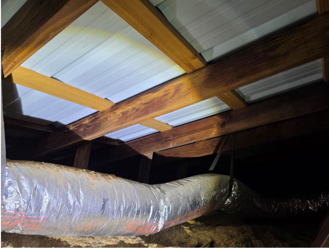
Photograph 5: Overview of the framing and covering of the roof
