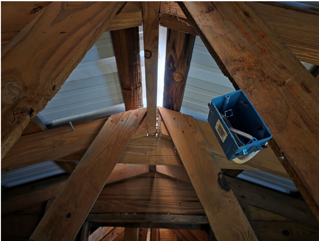
Photograph 6: Example of the ridge assembly and framing
