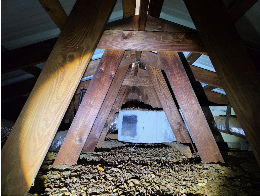
Photograph 3: Overview of the attic space
