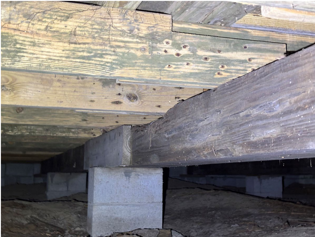
Photograph 8: Example of floor joists and beams supported by CMU piers
